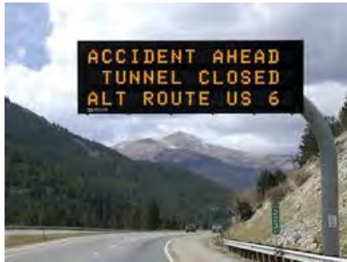
Figure 22 – Arterial Dynamic Message Sign
