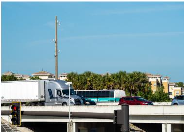
Roadside equipment: A single pole can support multiple ITS devices, including a CCTV camera, traffic sensors, and a control box. There is also room to mount equipment to communicate with connected vehicles.
