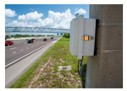
Connected vehicles: With the advent of connected vehicles, FDOT is deploying devices to communicate with passing cars, trucks, and buses. These devices connect to the ITS network and exchange data with the RTMC.
