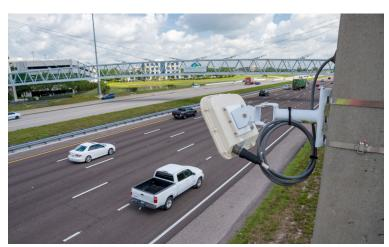
► Traffic detectors: More than 391 detectors use microwave or radar technology to determine the current speed and volume of traffic on monitored roadways. This helps detect slowdowns that can indicate incidents.
