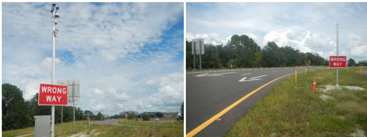
Figure 1: Recent installation along Interstate 4 at Lake Mary Boulevard (Exit 98) in Seminole County, FL
