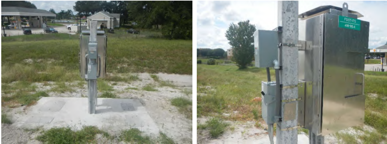
Figure 6: Type 336S local hub w/ concrete pad (left) | Local hub informational placard (right).
