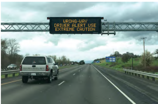
Warn right-way drivers on system-integrated overhead dynamic message boards
