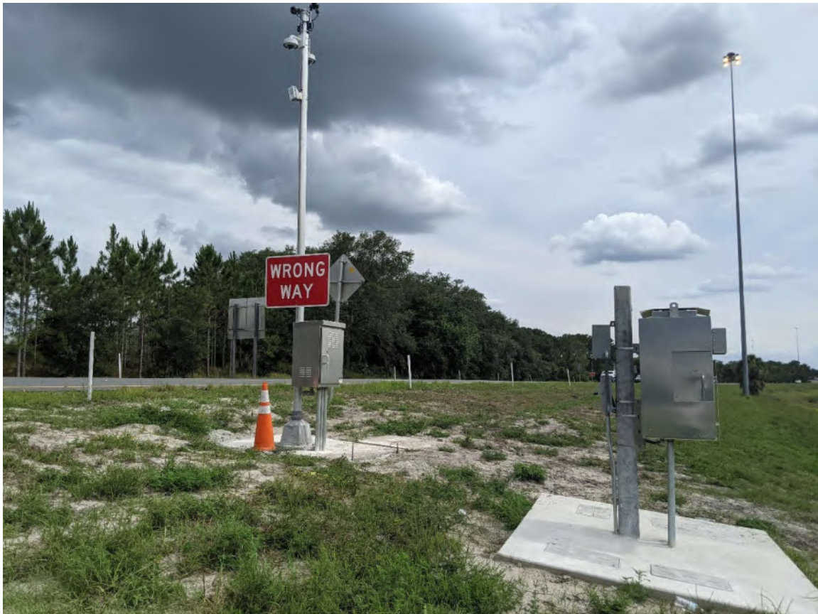
Figure 4: WWDS deployment w/ vehicle detection system, highlighted sign assembly, and local hub cabinet.
