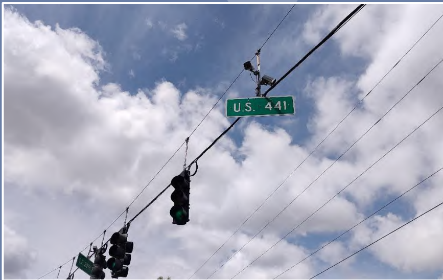
Span wire intersection with microwave radar sensors installed using mounting assembly attached to the catenary and messenger wires. (Marion County)
