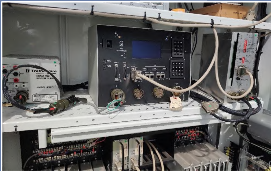
Q-Free (formerly Intelight) XN-2 ATC controller unit, TS-2, Type 2 model, operated as Type 1 ("A" connector only). (Lake County)
