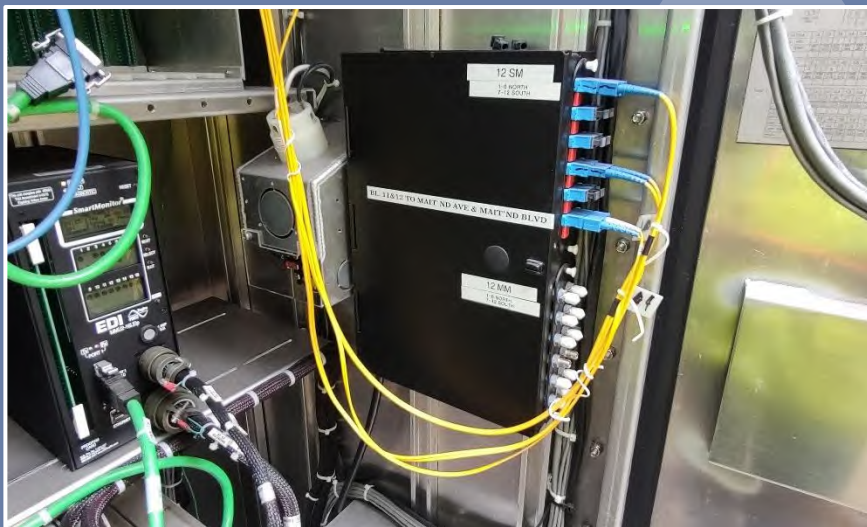
Fiber optic patch panel installed in controller cabinet assembly with two (2) fully terminated twelve-count connector panels. (City of Orlando)
