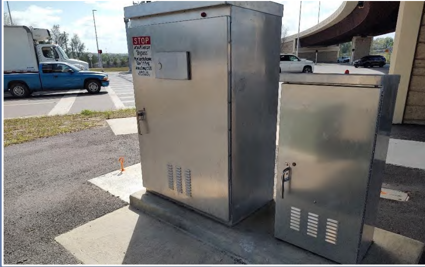
NEMA Type 6 controller cabinet assembly with stand-alone UPS cabinet on shared concrete base (foundation) with generator security anchor. (Lake County)
