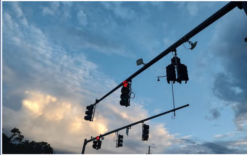
Multiple microwave radar sensors installed on mast arm assemblies on the near side of the intersection for stop bar detection. (Volusia County)
