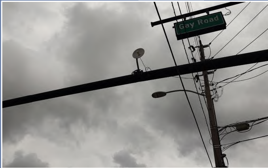
Dish-style point-to-point wireless radio installed on mast arm structure. (City of Orlando)
