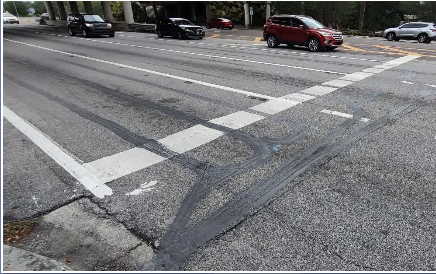
Type F inductive loops installed forty feet (40') in length with loop lead-in cuts. (City of Maitland)
