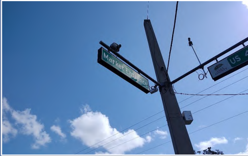
Hybrid video-radar unit installed on cantilevered mounting arm attached to the concrete strain pole at a span wire intersection. ( Lake County )
