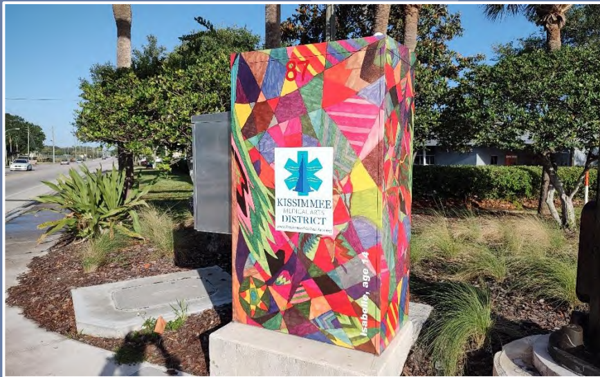
“Piggyback” UPS cabinet attached to the exterior side wall of the NEMA Type 6 controller cabinet assembly; some agencies may elect to wrap cabinet exteriors to match local aesthetic requirements. (Osceola County)
