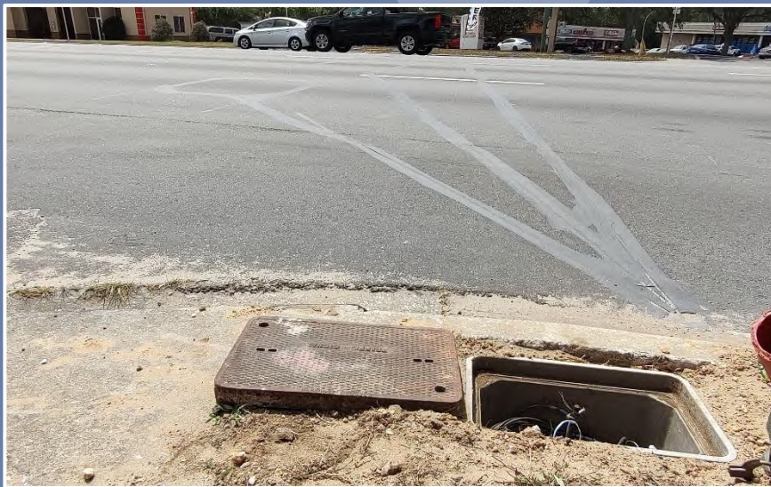
Loop lead-in wires for advanced detection cut in asphalt pavement surface to homerun pull box. (Marion County)
